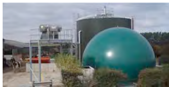
Digester and gas storage tank, Copys Green Farm. Courtesy of Farming Futures
