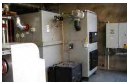
Boiler room at Carwood Close. 320kW biomass boiler. Courtesy of Econergy
