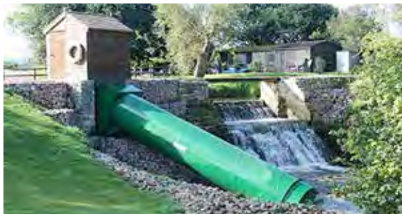
Archimedes screw and generator housing. Courtesy of Potenergy
