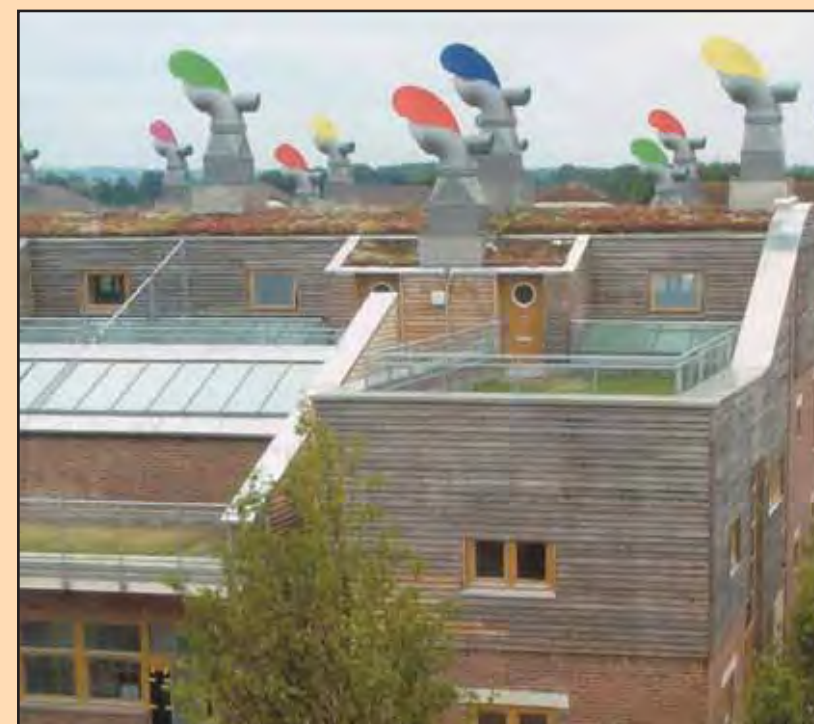
Chimneys can function as flues and/or as ventilation ducts.
