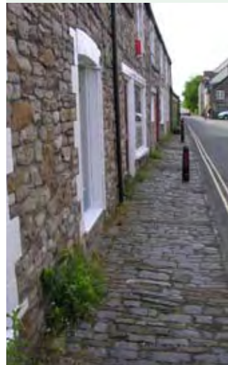
Traditional stone kerbs and sets to foot-ways should be retained. Avoid use of concrete kerbs or edging.
