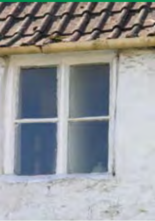
Simple symmetrical casement window.
