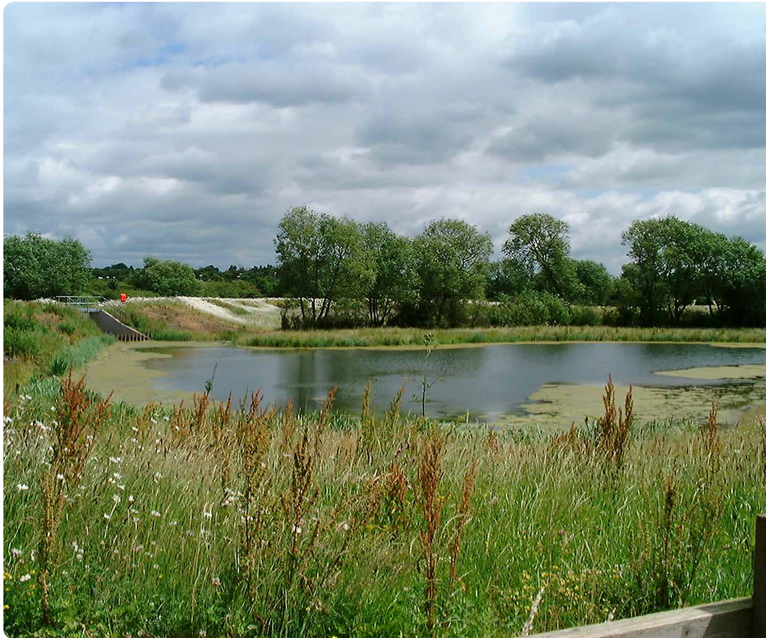
Figure 19: Detention Basin – Emersons Green
