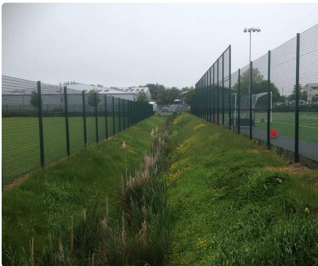
Figure 8: Swale at Abbeywood Community School (Stoke Gifford)
