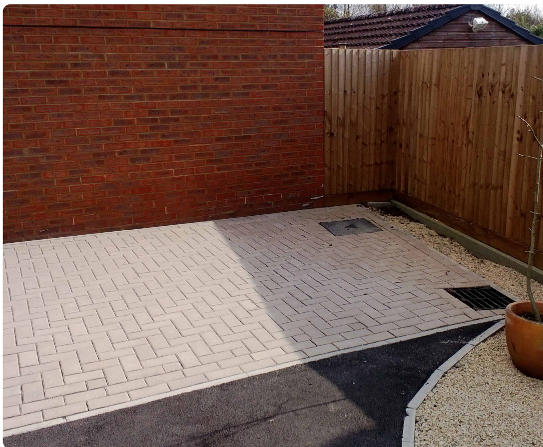
Figure 14: Example of Permeable Paving
