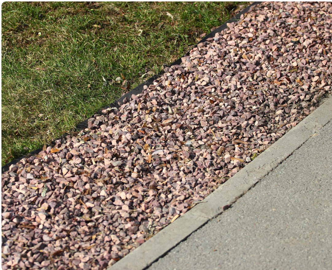
Figure 17: Example of a Filter Drain / Strip
