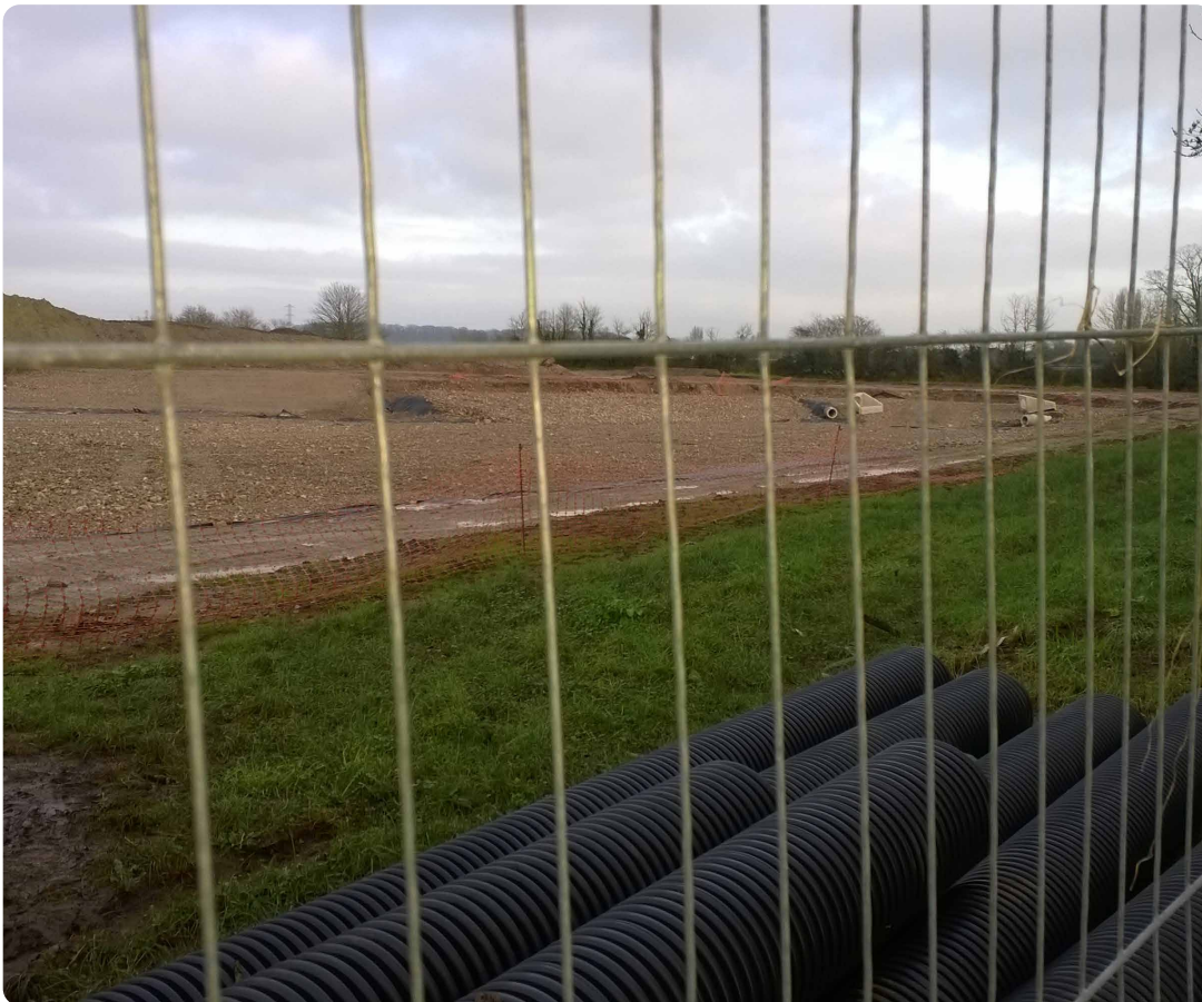
Figure 21: SuDS attenuation feature under construction
