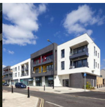
Balcony and amenity space, Holland.
