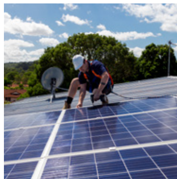
Solar panels being fitted to a house roof.
