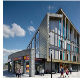
Keynsham Civic Centre - Mixed Use Development.
