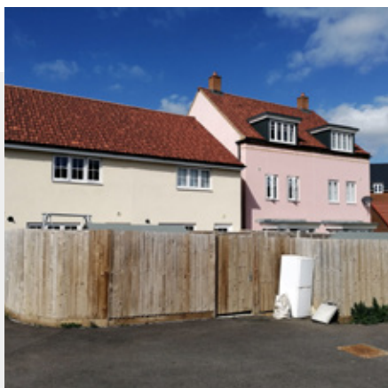
Rubbish dumped in poorly maintained rear parking court.
