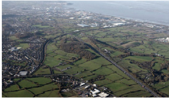
Avonmouth Severnside Enterprise Area flood defence project.
