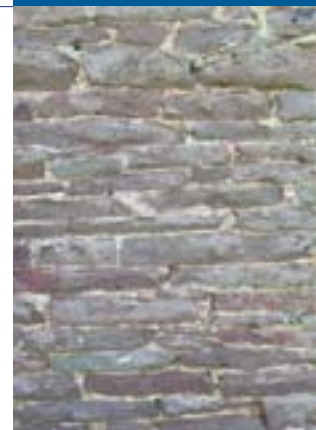
Wall pointed with lime mortar. The mortar is old but not failing and does not need to be replaced.
