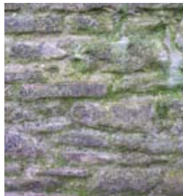
Manure has been applied to the new lime mortar pointing in order to encourage algae growth which will 'age' the appearance of the new pointing.
