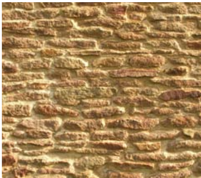
New lime mortar pointing correctly finished. The mortar is slightly recessed from the face of the stone, and brushed and tamped back to create an open texture and expose the aggregate.
