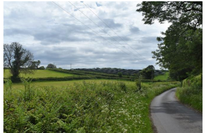
Existing Band C solar farm at Tower Hill Farm in LCA G18.
