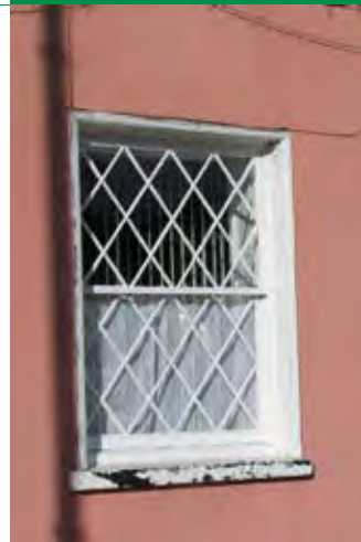
Diagonal glazing bar sash window.
