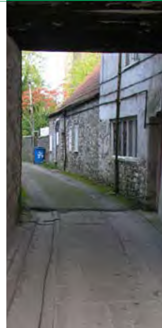
Archway to rear of burgage plot with its range of buildings.
