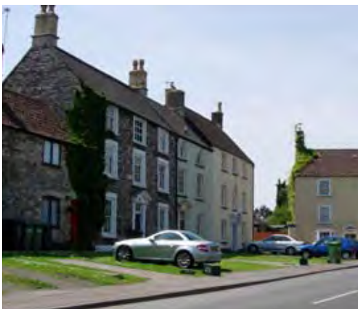
The attractive group of Georgian terrace houses by the bend close off the view.
