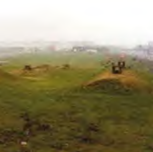
Air Raid Shelters - Filton
