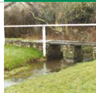
Stone footbridge - Station Road, Yate
