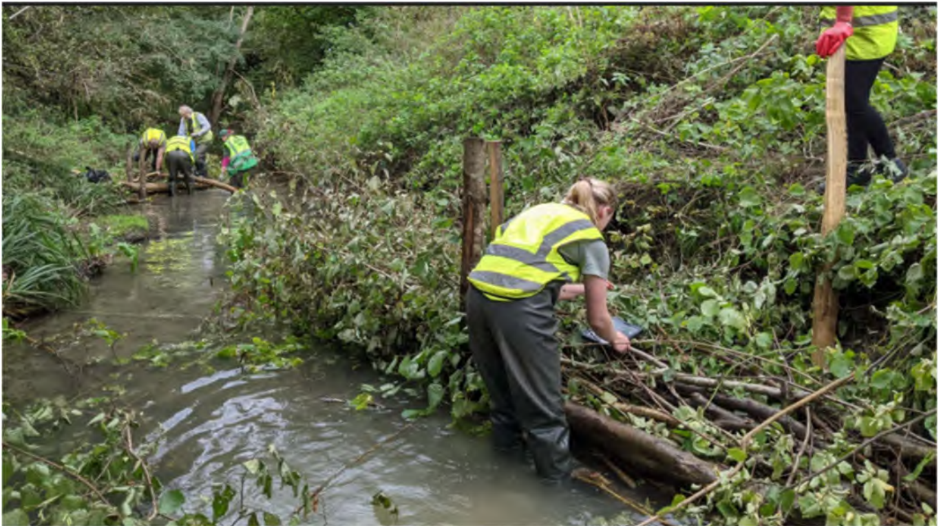
Source: South Gloucestershire Council, Environment and Community Services
