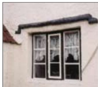
Render correctly swept over the head of the window
