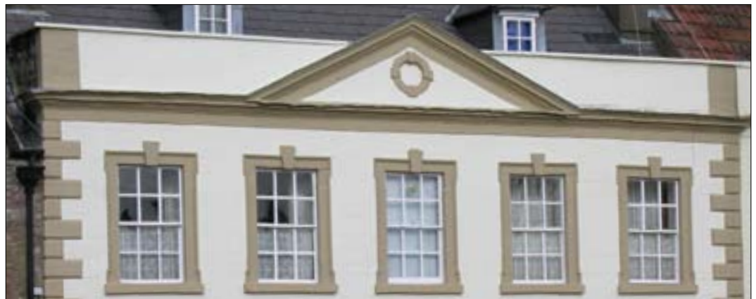
Stone quoins correctly pronounced from render
