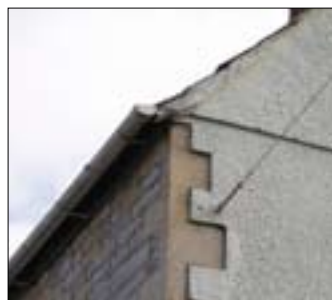
Render incorrectly pronounced beyond stone quoins
