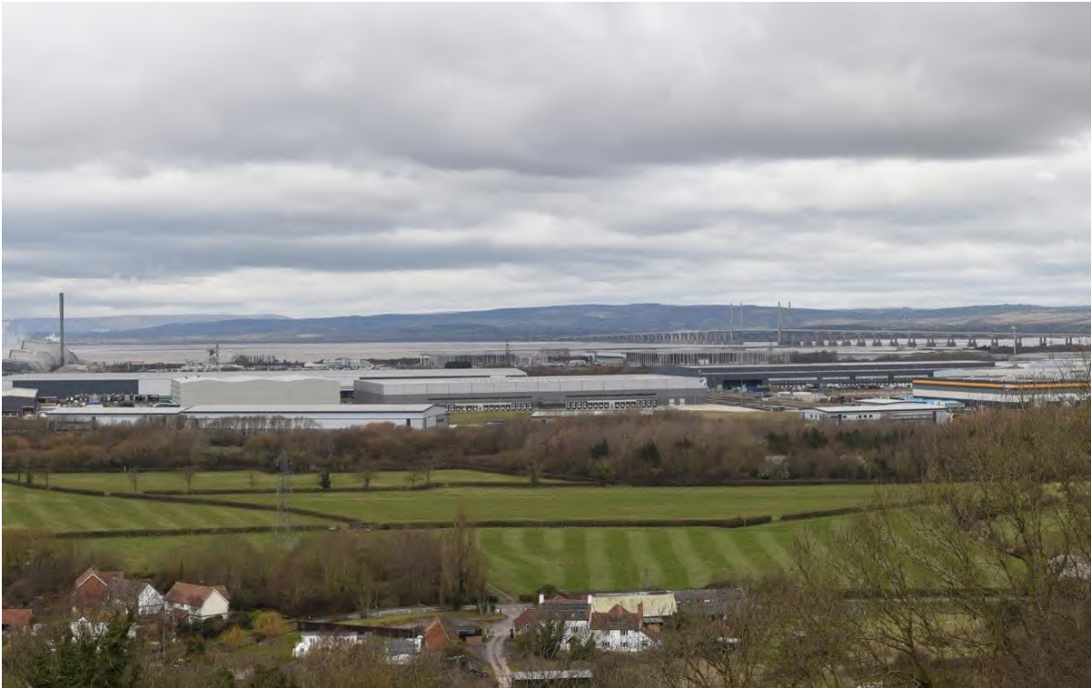
Photo 4: View west from Spaniorum Hill across industrial infrastructure and warehouses at Severnsde Works and Western Distribution Park
