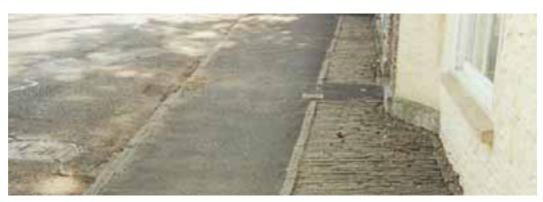
Originally quarried locally the characteristic pennant stone kerbs & setts to foot-ways should be retained. The use of concrete kerbs or edging is considered harmful.
