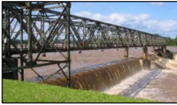
Figure 5: Hydropower Energy Generator
