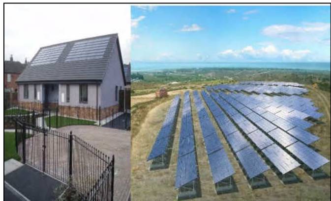
Figure 20: A Rooftop Solar Array
