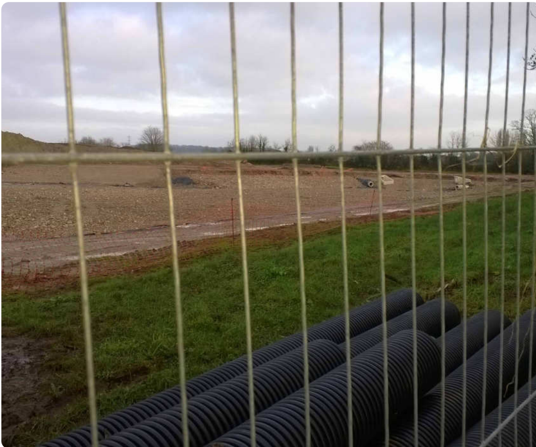
Figure 21: SuDS attenuation feature under construction
