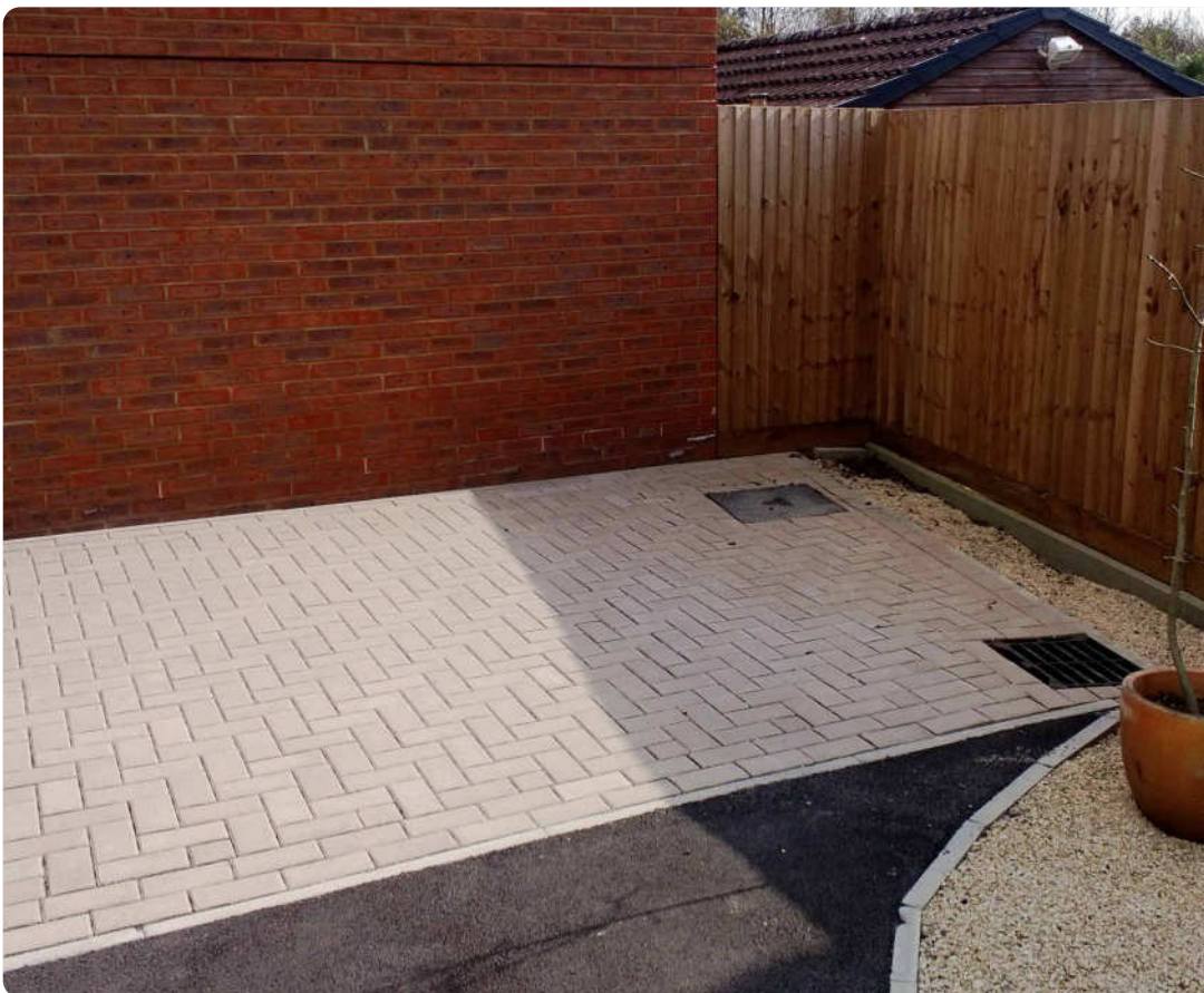
Figure 14: Example of Permeable Paving
