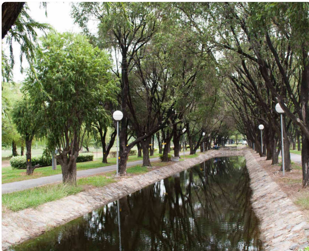
Figure 15: Example of a swale with walkway beside
