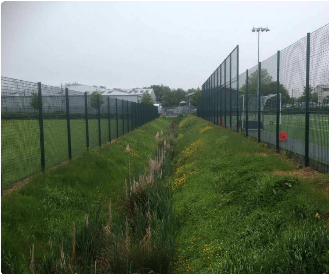
Figure 8: Swale at Abbeywood Community School (Stoke Gifford)
