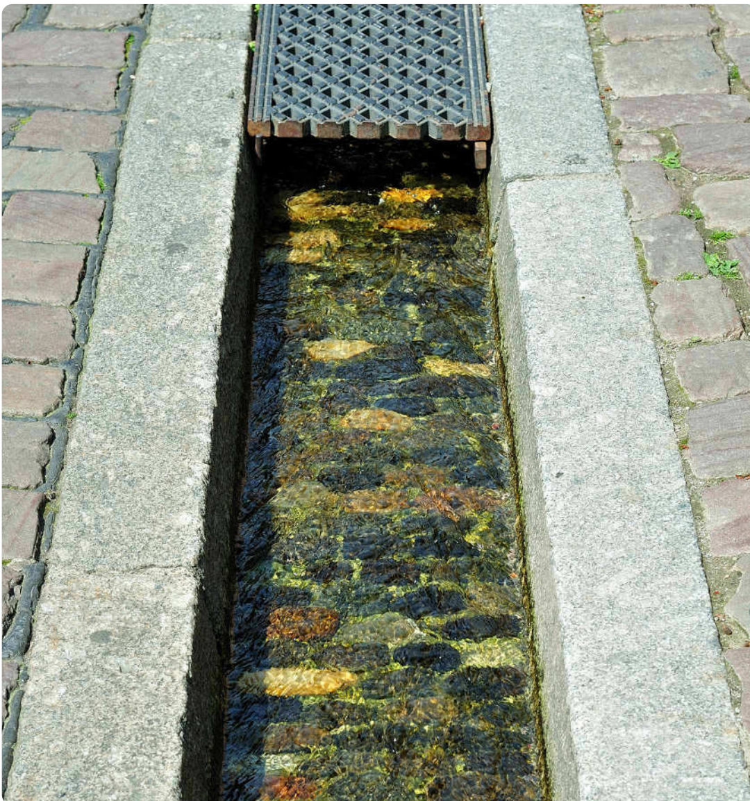
Figure 16: Example of a Typical Rill Channel
