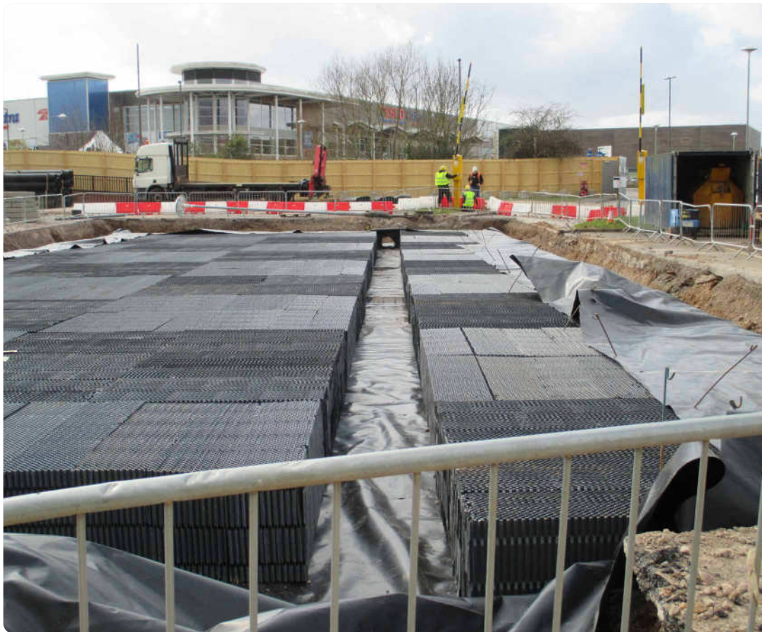
Figure 20: Geocellular Storage Crate System under construction in Yate
