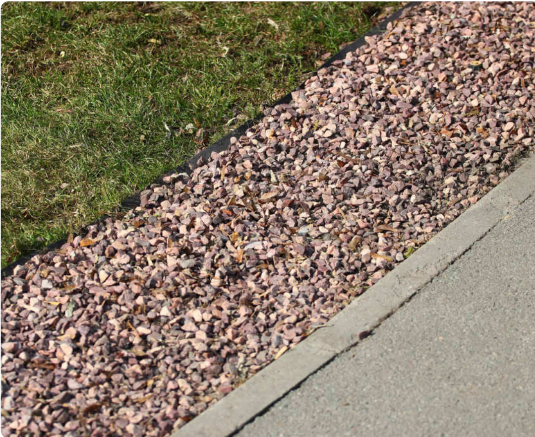
Figure 17: Example of a Filter Drain / Strip
