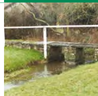
Stone footbridge - Station Road, Yate
