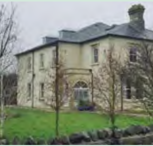
Queens Lodge - New Passage
