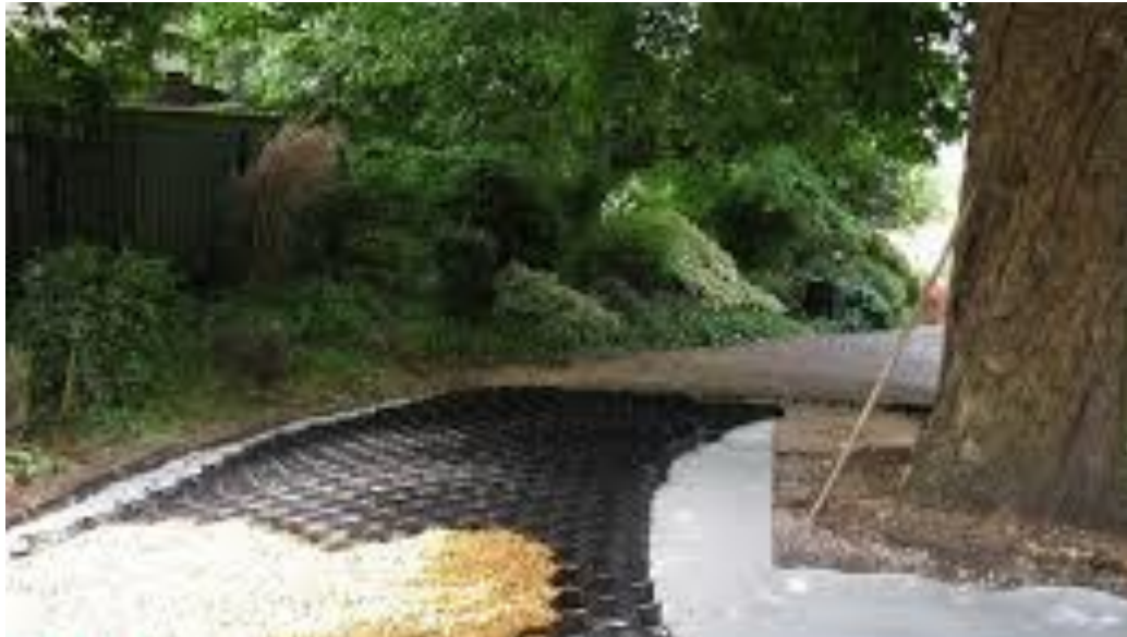
Example of no-dig construction next to a mature tree.
