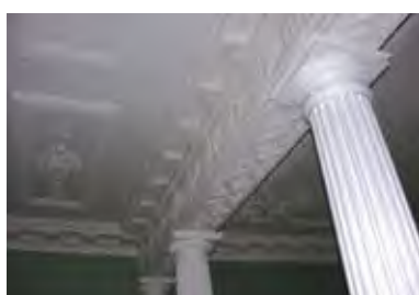
Early 19th century plasterwork
