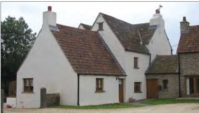
Hallen Farm before and after restoration
