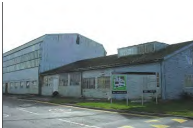
Barrage Balloon Workshop, Pucklechurch – grade II
