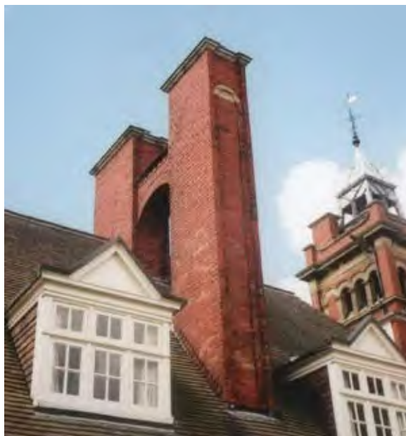
Chimney stack at Old Cottage Hospital Almondsbury
