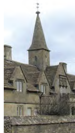
Crispe Almshouses, Marshfield – grade II
