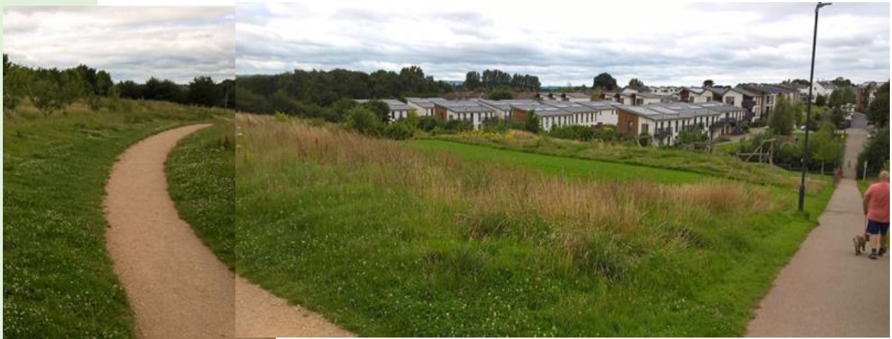
Hanham Hall POS; footpath/cycleway in coloured asphalt, right, provides a durable surface suitable for all users, connecting to the Bristol-Bath cycletrack. Bound gravel surfaced path to the left, used as a secondary route through the wildflower meadow area.
