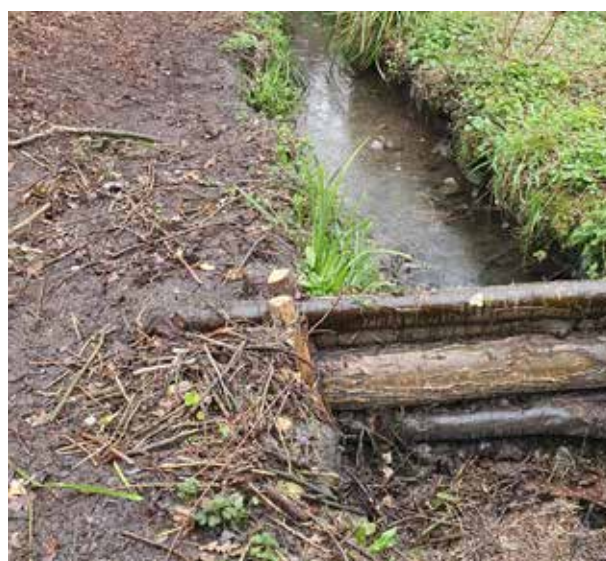
A 'leaky dam' to slow the flow on Stoke Brook to help reduce flood risk on the main Bristol Frome river.
