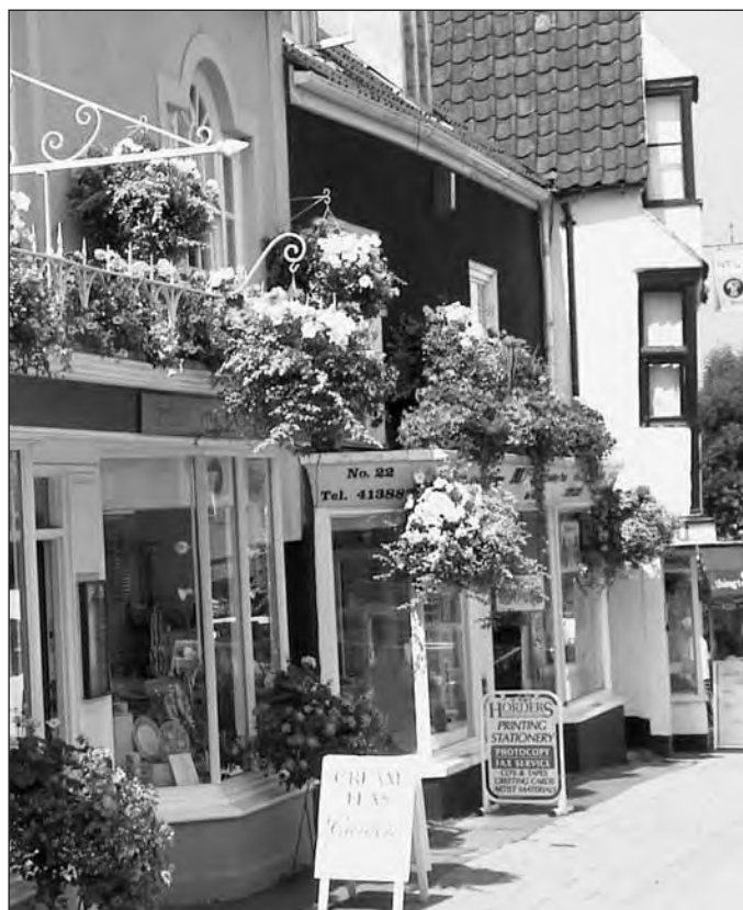
The attractive shop frontages contribute greatly to the character of the High Street - but careful management of advertisements and forecourts is required.
