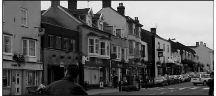
Shop front details are critical
