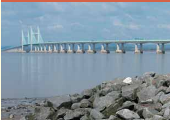
Second Severn Crossing
