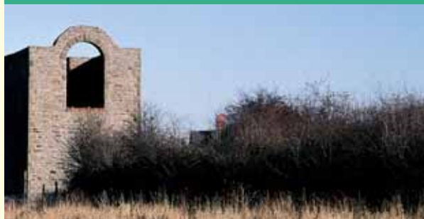
Church Farm Deep Engine House
