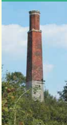
Brandy Bottom Chimney
