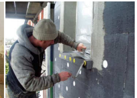
Photo of window install in Enerphit retrofit (© Passivehouseplus)
