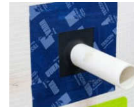
Airtightness grommets need to be used so that service penetrations do not increase air permeability
