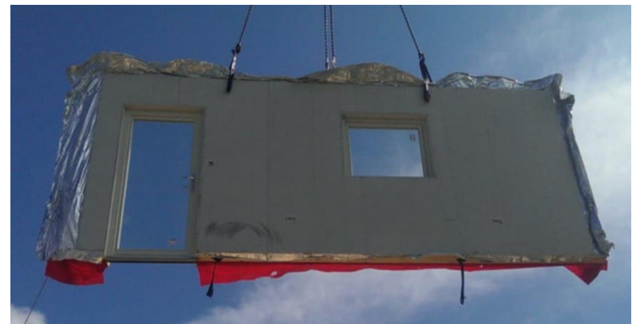
A closed-panel timber frame, manufactured off-site with insulation, window and door frame included (© Vision Development).
