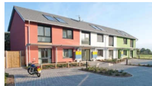
Wimbish Passivhaus certified. © Hastoe Housing Association.
