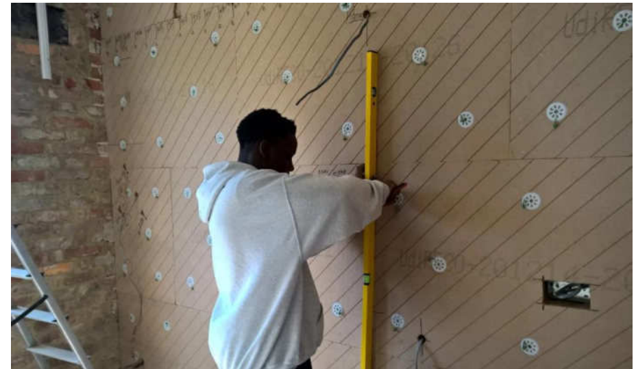
Installation of wood fibre insulation boards internally (© Back to Earth & ASBP)
