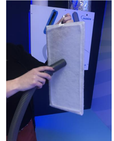
MVHR filters are easy to remove and clean, clean filters improve energy efficiency
