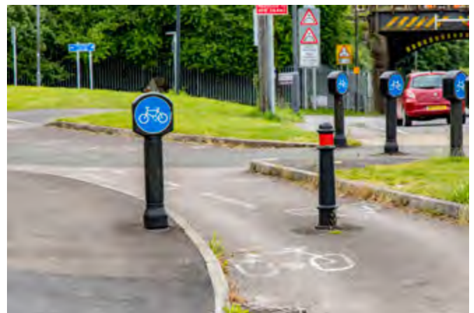
10. Existing cycle lanes on Hatchet Road. Courtesy Rich McD
