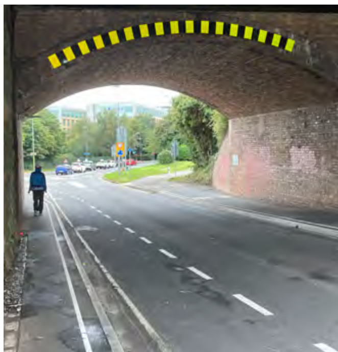
7. Brierly Furlong Underpass
