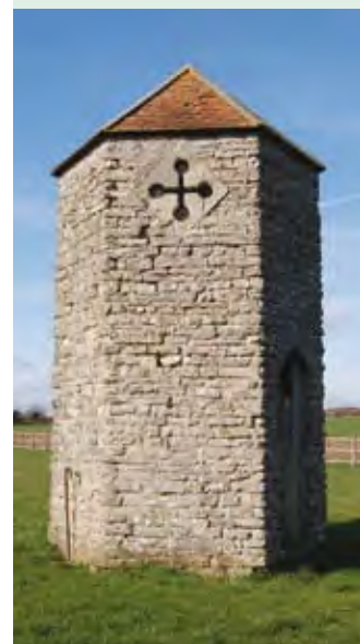
The Well House at Siston Court.
