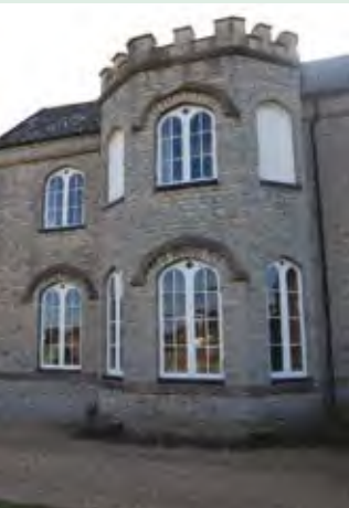
The Grange (Circa 19th Century). - The former nurseryman's home in the Gothick Style.
