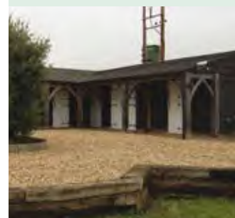
A development of stables within the curtilage of Siston Court with its associated landscaping has failed to respect character of the area. Similar developments should be resisted due to harm to the green setting of Siston Court.
