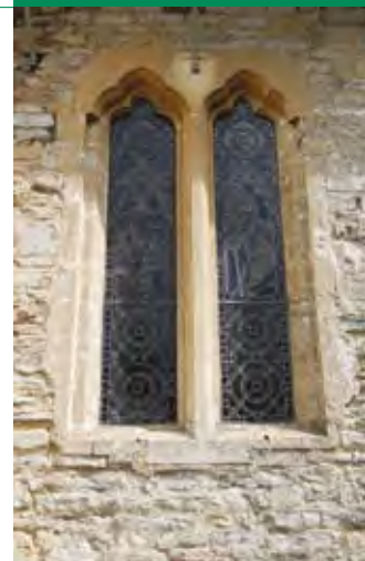
Trefoil headed lancet windows at St Anne's Church.
