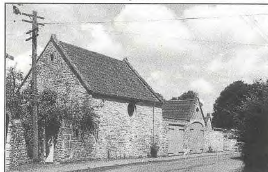
Stone buildings and boundary walls adjoining Upton House
