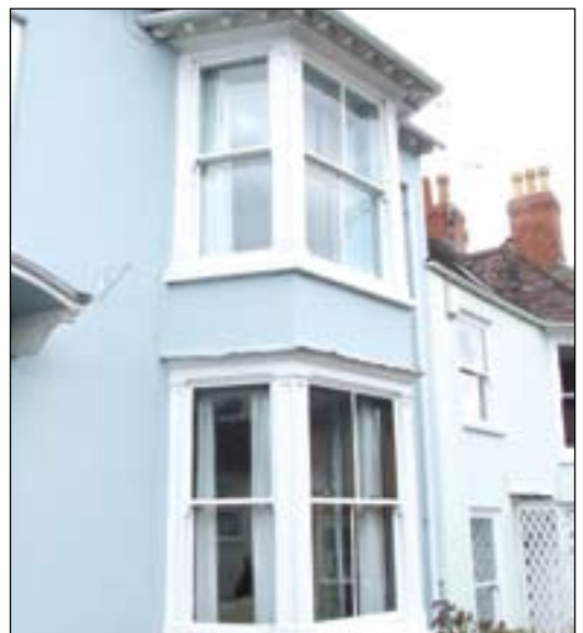
Victorian sashes with large panes and horns.
