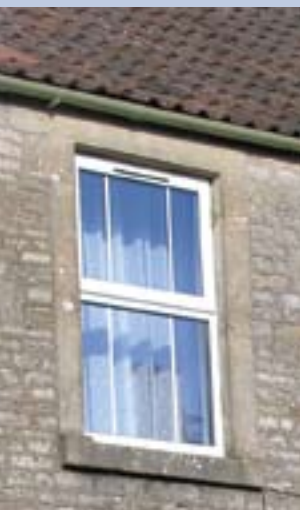
Modern top hung uPVC window with stick-on glazing bars and trickle vent, and 'storm proof' design.
