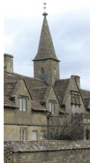
Crispe Almshouses, Marshfield – grade II
