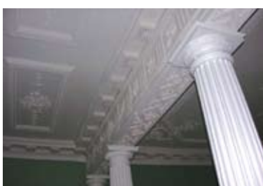
Early 19th century plasterwork
