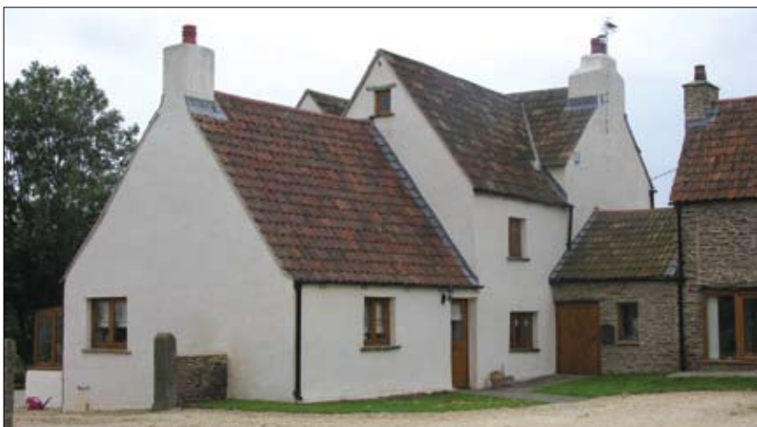
Hallen Farm before and after restoration
