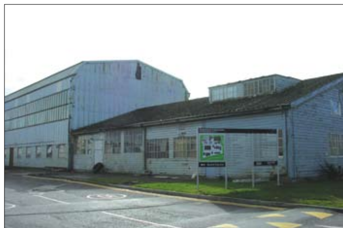
Barrage Balloon Workshop, Pucklechurch – grade II
