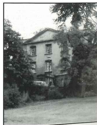
Warmley House overlooking the gardens.
