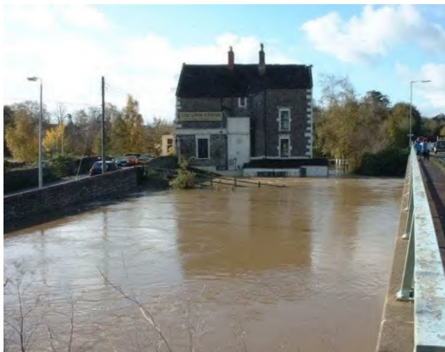
Figure 7 - Flooding at Keynsham Road
