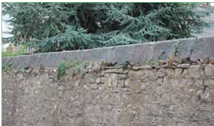
Traditional slag coping to wall top
