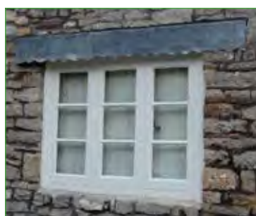
Traditional flush timber casement
