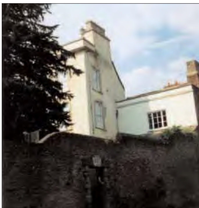
Hambrook House - partially hidden behind trees and boundary walls
