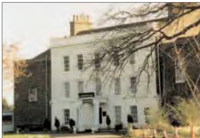
It is important that any alterations do not harm the historic character
