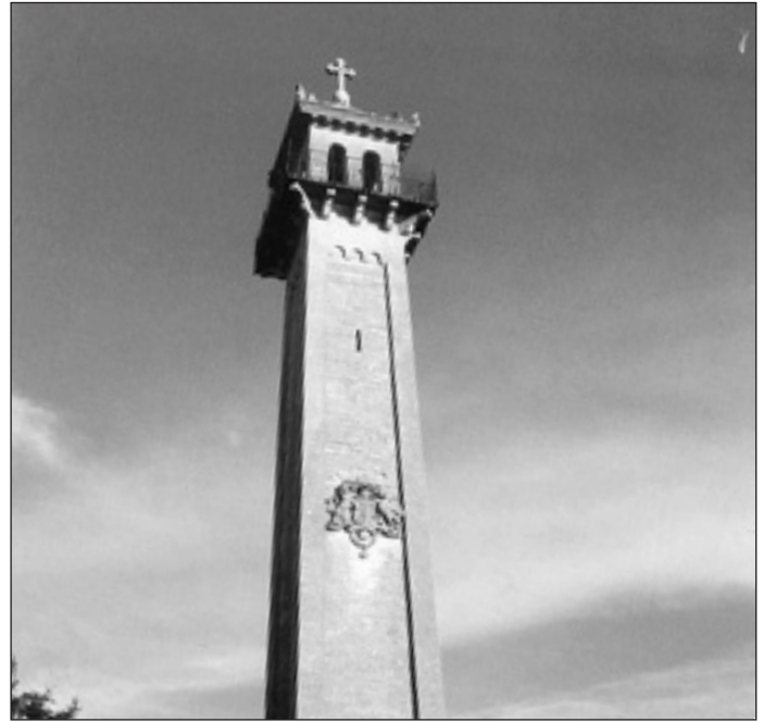
The Monument, an impressive structure, is in need of repair.
