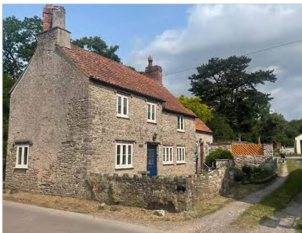
Lindum Cottage is a locally listed building. The historic tree belt to the north provides amenity value to this part of the Conservation Area
