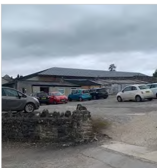
The car park would benefit from landscaping enhancements
