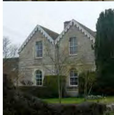
**Roofing:** Roofing materials are predominantly clay double roman and pan tiles, with natural Welsh slate found on some of the higher status houses. There are occasional instances of natural Cotswold stone tiles being used. Modern artificial slate and concrete tiles are being introduced as replacements to traditional roofing materials although these tend to diminish the traditional character of the area.
