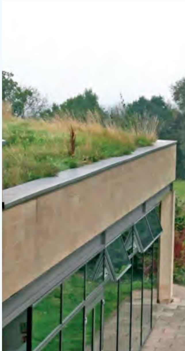
Wessex Water SuDS system
