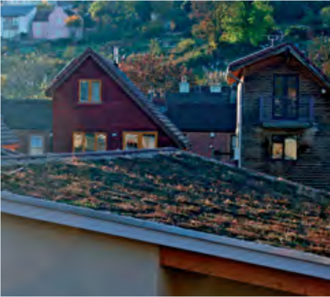
Ashley Vale green roof
