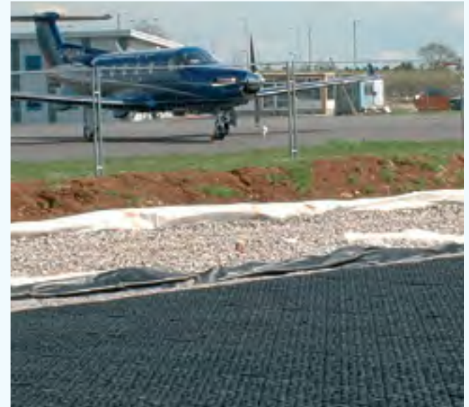
Bristol Airport Car Park permeable paving
