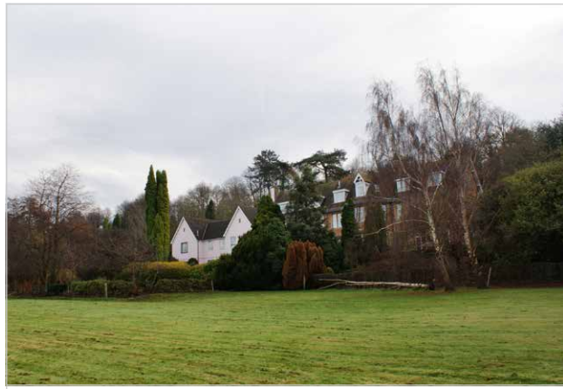
Extensive lawns to Glebe House form an important open space and setting to the church
