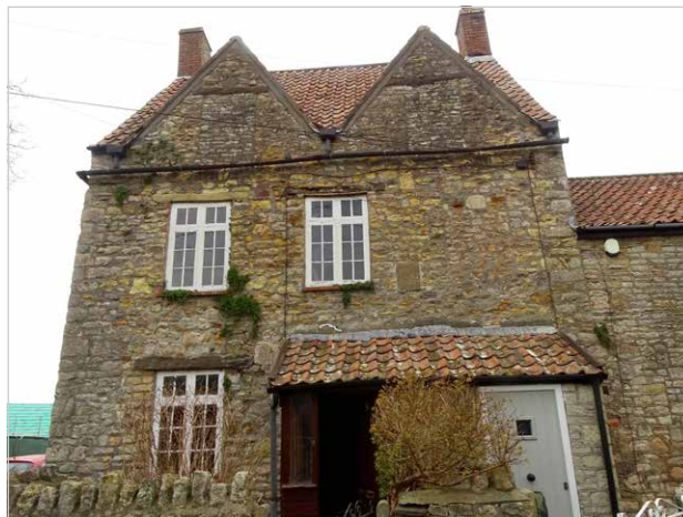
This house on Lower Court Road (grade II listed) is a good example of a seventeenth century gabled vernacular farmhouse
