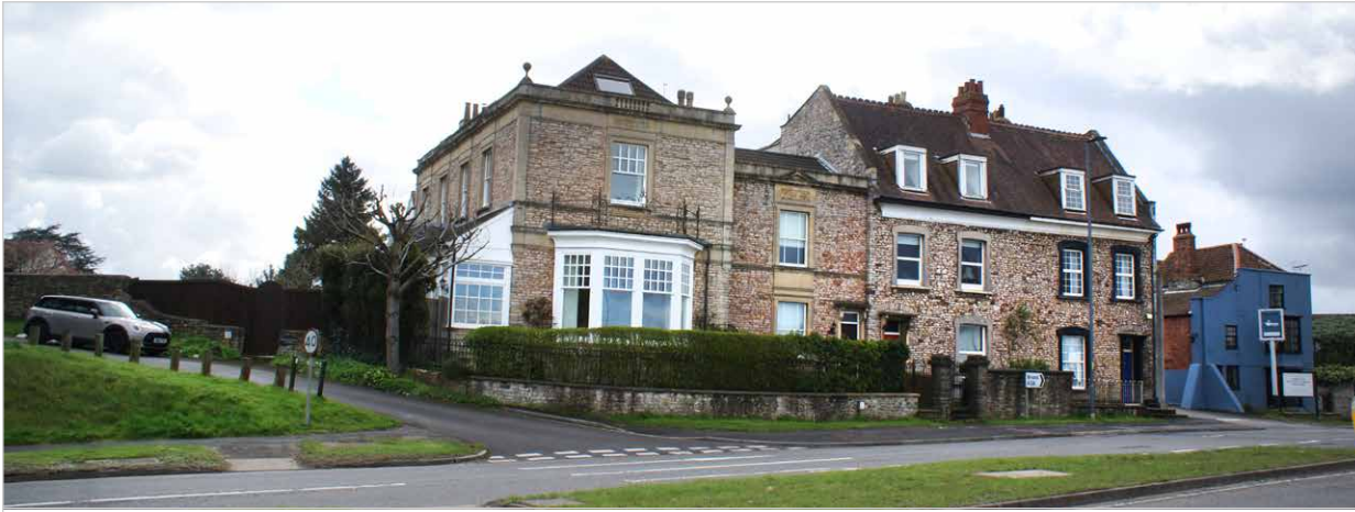
Polite buildings with classical detailing help define this part of the conservation area
