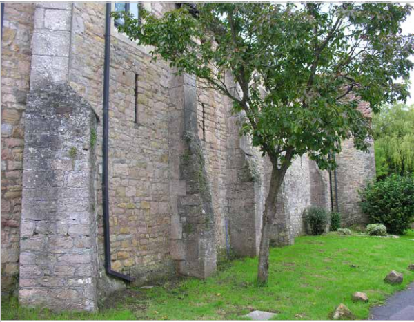
Court Farm Barn, with its distinctive buttressed walls, dates from at least the early sixteenth century. It is likely to have been built as a lodging range for the manorial complex of St Augustine's Abbey, before being converted and adapted for agricultural use
