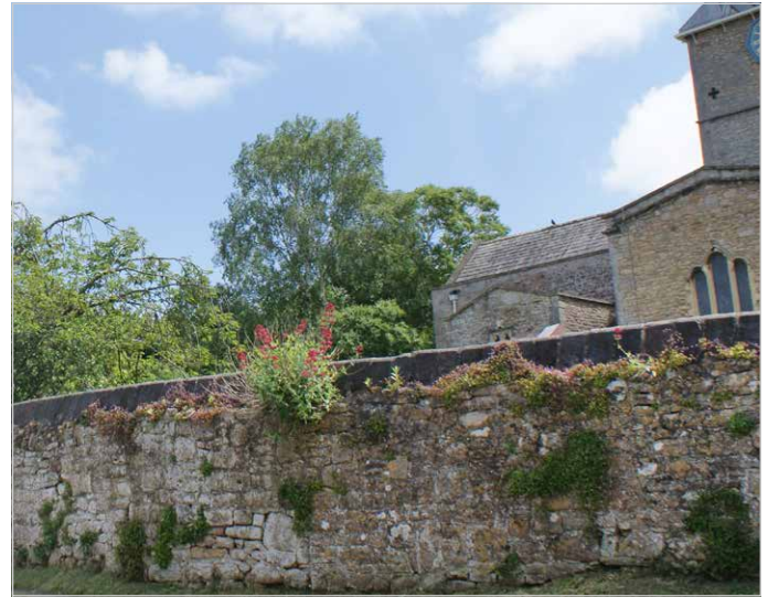
The wall to the church yard of St Mary's is topped with distinctive large black slag block copings, a product of the copper smelting of the South Gloucestershire and Bristol area in the eighteenth century
