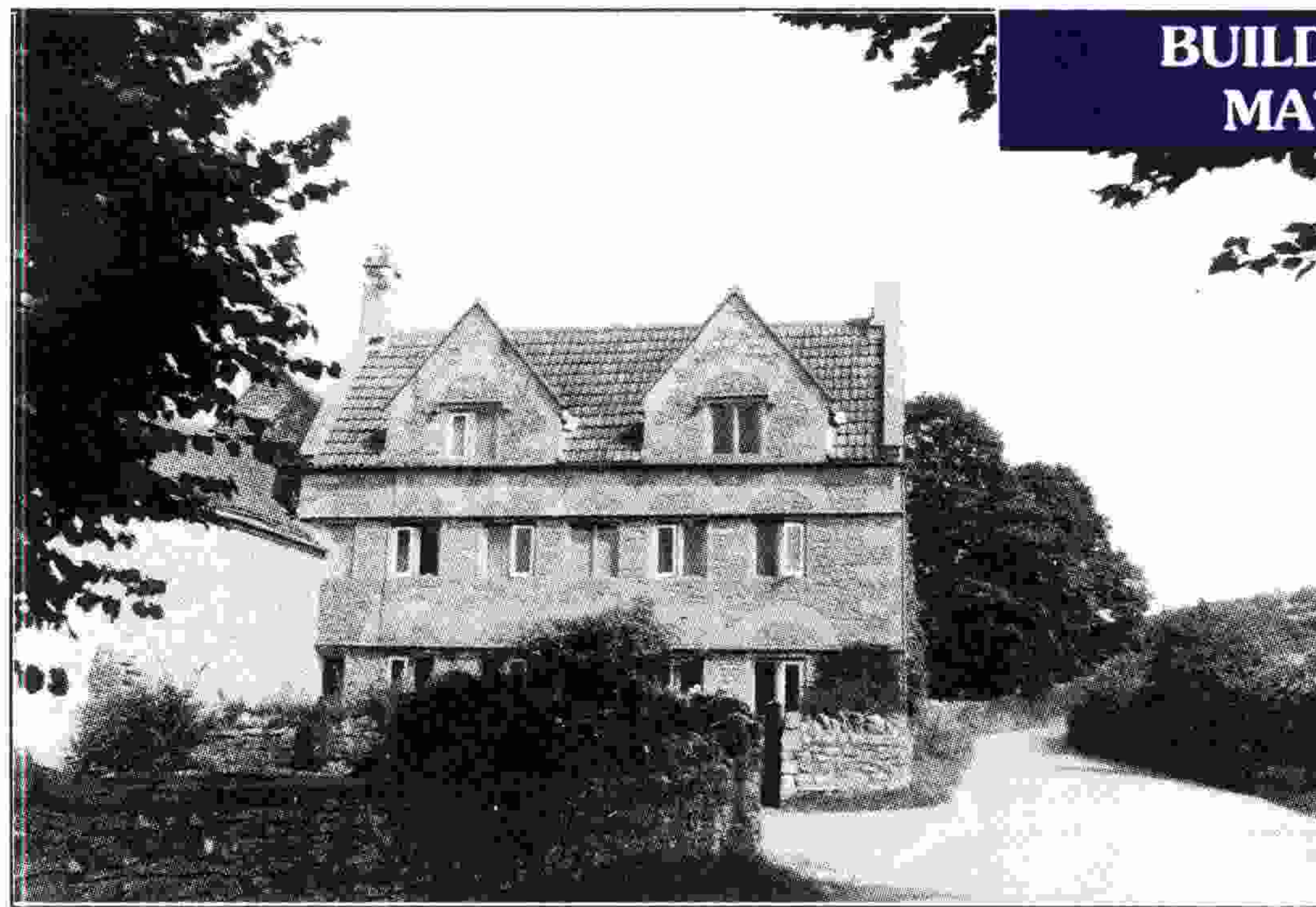
Brittons Farm located at right angles to the enclosed lane.
