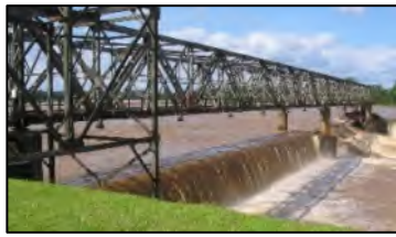
Figure 5: Hydropower Energy Generator
