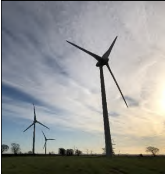
Figure 19: Earthcott Wind Farm - Alveston
