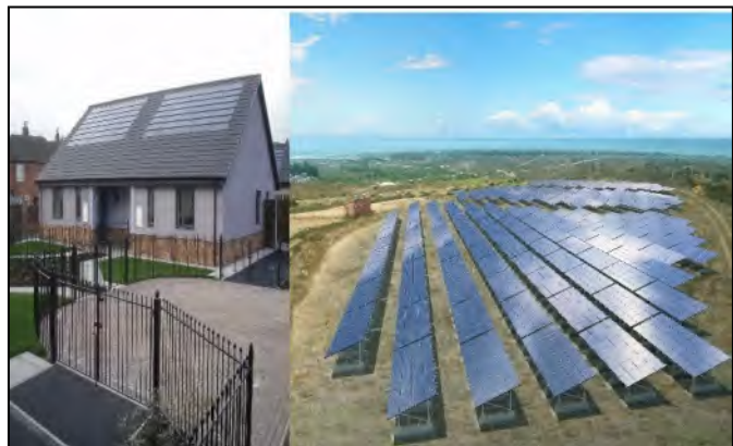
Figure 20: A Rooftop Solar Array
