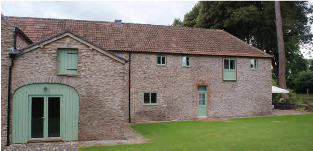
FIG.15 Note hay loft door above flat arch and also stable door to its right at first floor level. This approach to maintaining the openings and whether functional or not is considered to be an important part of what is a good example of a residential conversion of a former stable as it has retained the random nature of the openings in terms of positioning and scale
