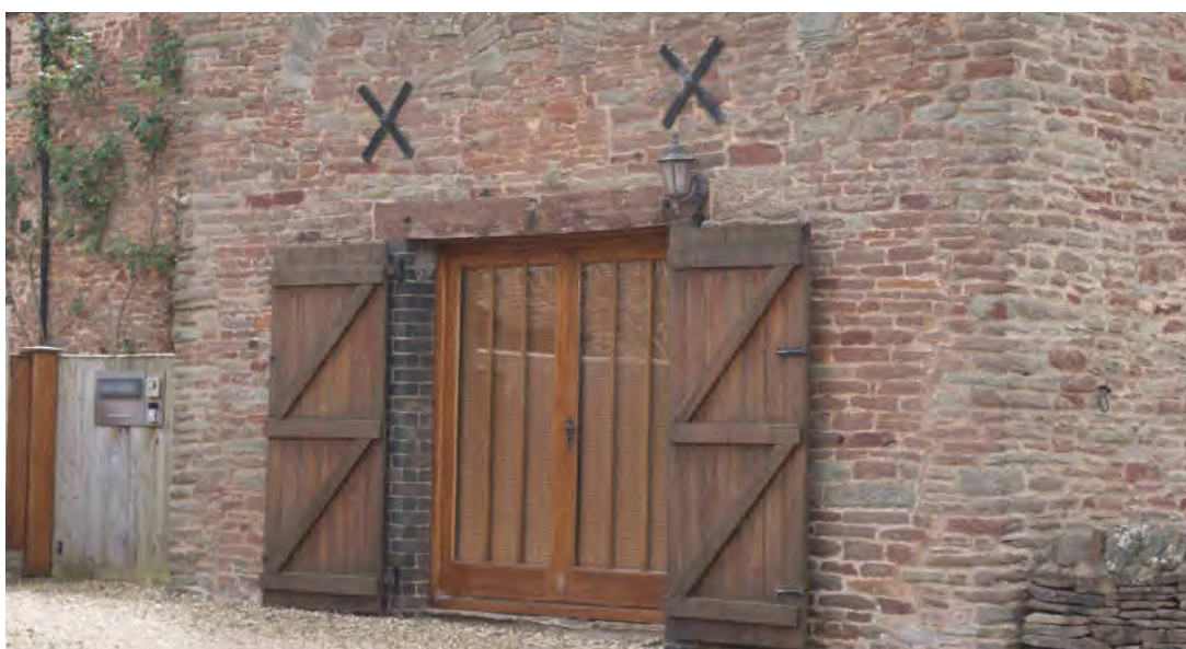
FIG.17 A good example of how to approach either an existing or new opening in terms of simple door design and use of shutters under an exposed timber lintel. The use of external shutters and blue engineering bricks to door reveals also add interest
