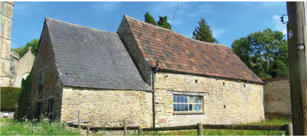
FIG.13 Two examples of barn conversions where the urge to insert new windows has been resisted which has maintain the existing opening only help retains the proportions and aesthetic character of the building
