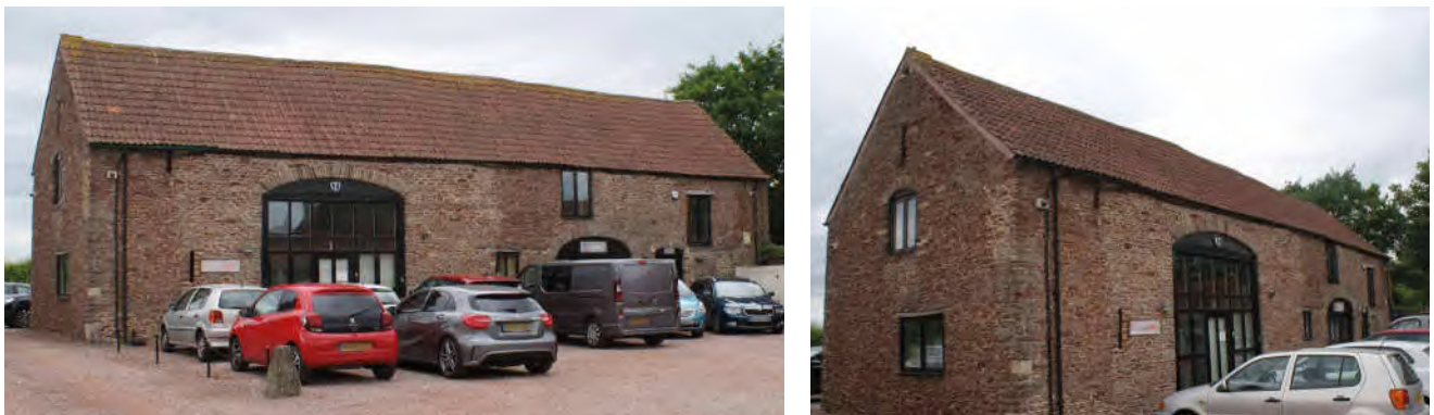
FIG.5 An example of a successful conversion of a traditional rural building and farmstead into a commercial use. Note the existing cart entrance and ventilation slots have been retained, as has the ad-hoc nature of the openings to the front elevation
