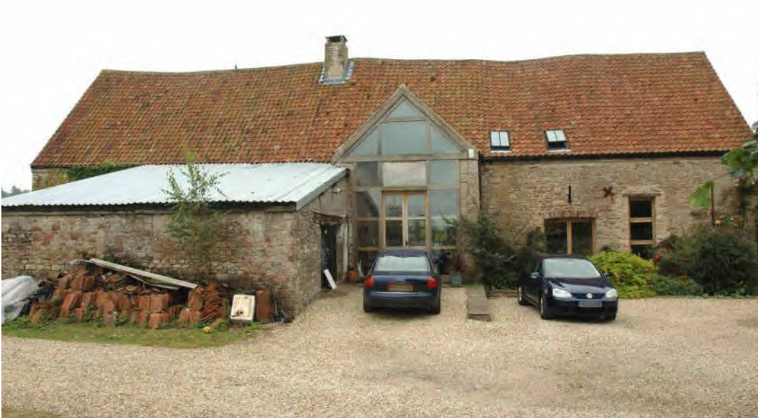
FIG.14 Here to proportions of the cart entrance to the central gabled projecting porch have been retained, as have the other existing openings
