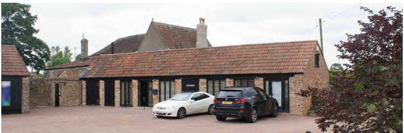
FIG.6 This commercial office is a converted shelter-shed. The previous use is still articulated with the rhythm of the bays and stone columns, as well as the roof plane remaining unbroken
