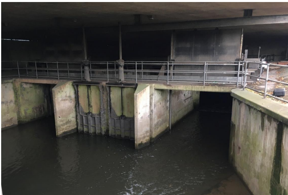
Figure 13 Northern Stormwater Interceptor at Eastville.
