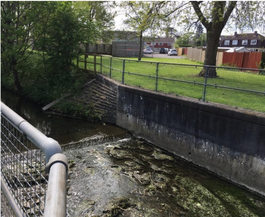
Figure 18 Fish barriers on the Frome prevent native fish moving up and down the river
