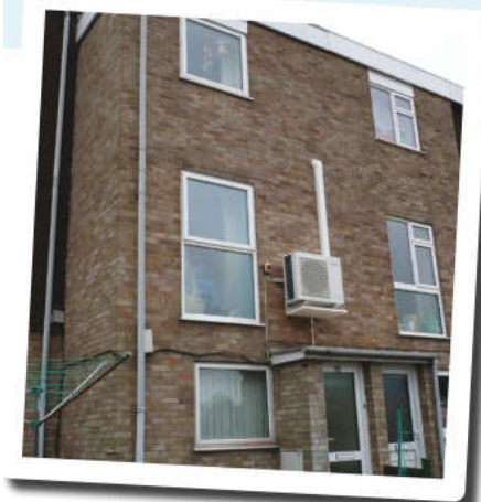
Figure 11: Air to Air Heat Pump
