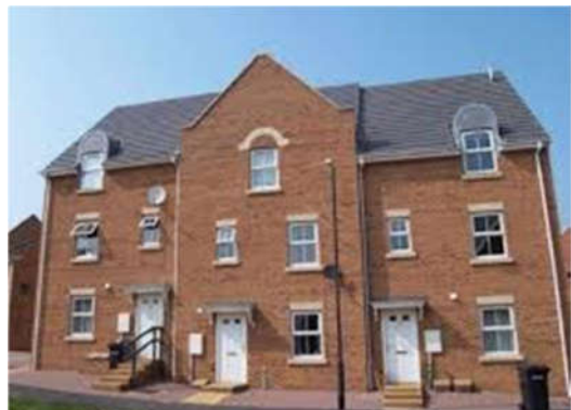
Figure 18: A House in Multiple Occupation
