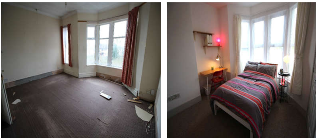
Figure 20: Front bedroom before and after refurbishment
