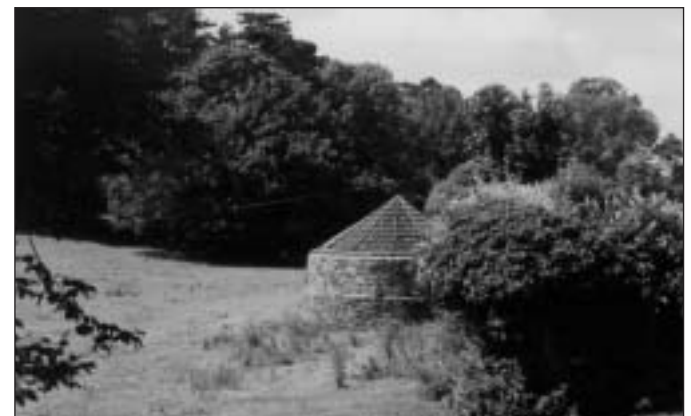
The railway air shaft - set within the landscape
