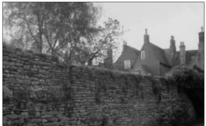
Stone boundary wall to Burgage plot
