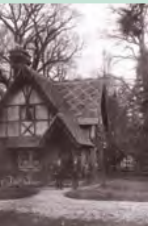
Gate Lodge to Frenchay Park.
