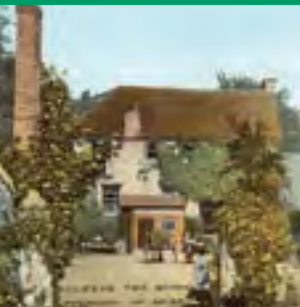
Cleeve Mill - converted for use as a tea garden. Now a private dwelling.
