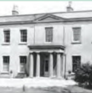
Newlands - now demolished. Its garden walls & outbuildings remain.
