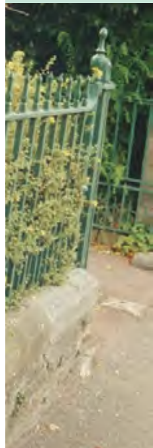
Stone wall and railings.
