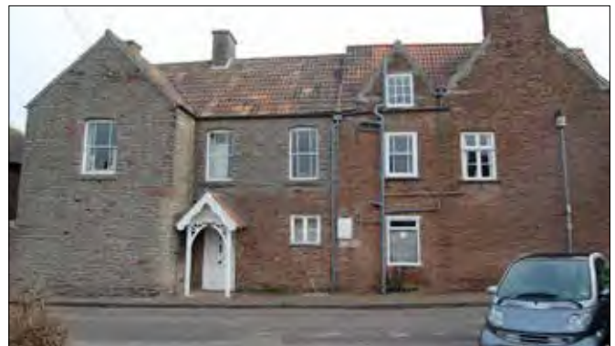
17th century The Gables with red and grey pennant stone showing different phases of construction.
