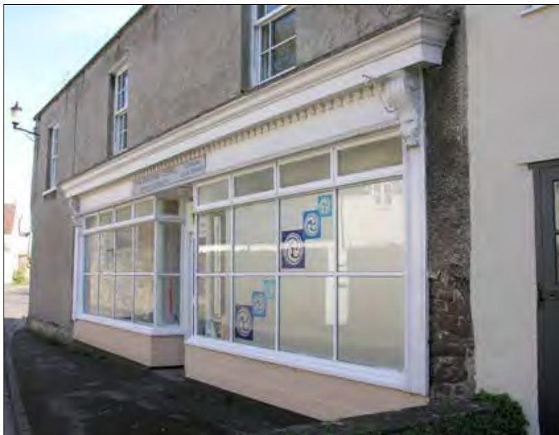
The ornate corbel brackets, fascia and cornice of a 19th century shopfront survive on this building in the High Street.
