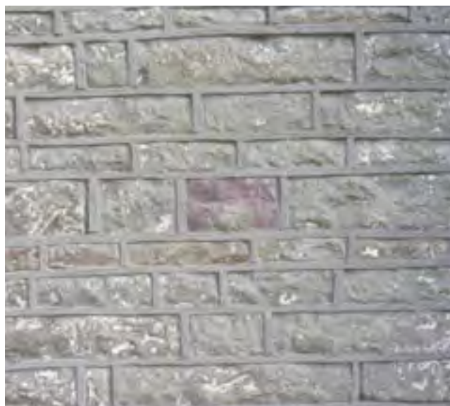
Incorrect ribbon pointing in hard cement. The pointing is finished proud of the stones, creating a harsh and untraditional appearance.
