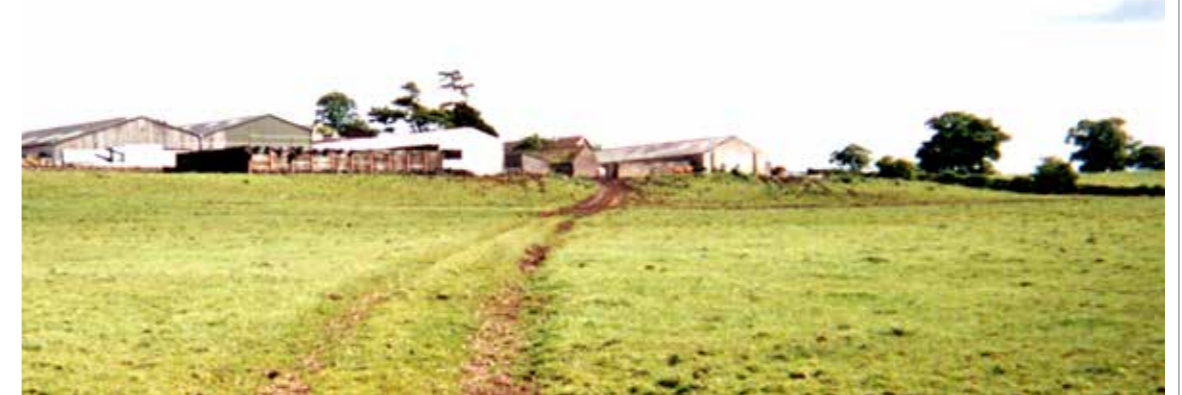
4 View south to Bagstone Court Farm - modern agricultural buildings replace the old cattle yard. These buildings are evident in views from the M5.
