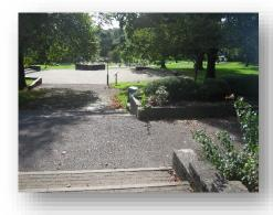
A large number of paths are in poor condition, with cracks, bumps and surface breaks due to tree root heave, weathering, and wear and tear. There are also crossfalls on many paths which are greater than the 1:50 maximum standard. The poor state of the paths and crossfalls restrict access for some people.
