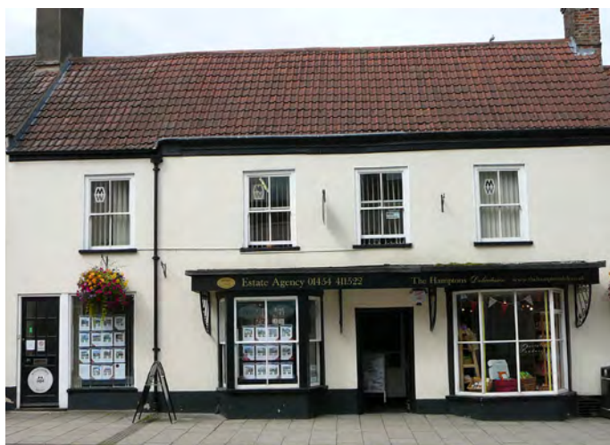
A mid-late 18 th century, Grade II listed building with later 19 th century bay windows under a continuous roof. To the left is the entrance to the upper floors.
