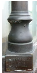
20 th century enhancements in shop design saw the introduction of curved glazing, tiling and the use of bronze in the construction of shopfronts.
