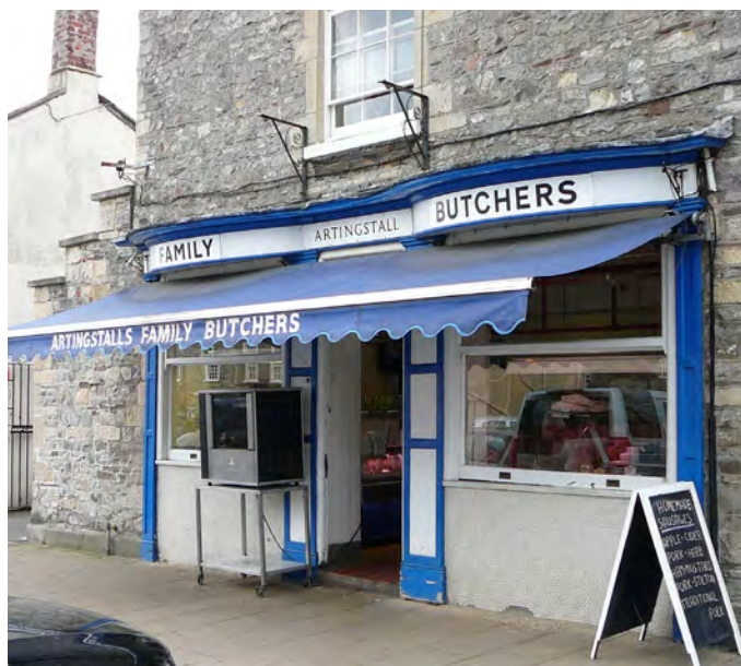
A good mid-19 th century butchers shopfront in a Grade II listed building. The original bow windows have been removed and replaced with sash widows but the cornice, pilasters and frieze survive.
