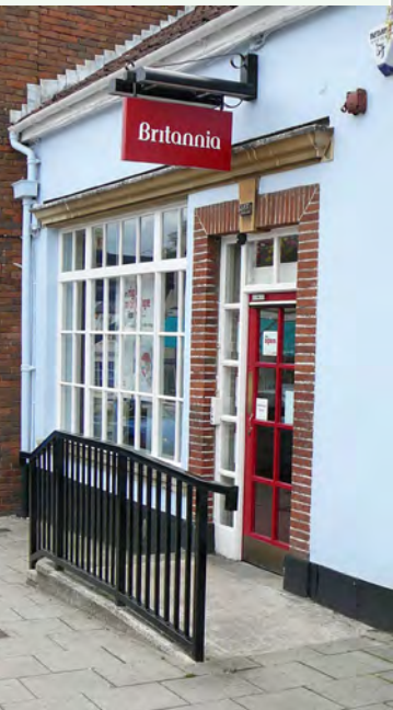
A typical level access to a shopfront where footpath width permits. Re-grading the footpath can sometimes avoid the need for a ramps.
