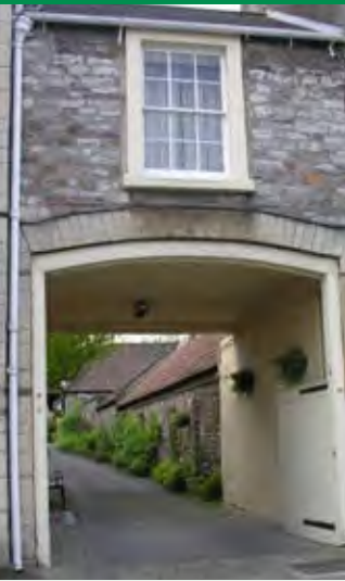
The archways to the rear plots give glimpses out from the main street which contribute to a sense of mystery.
